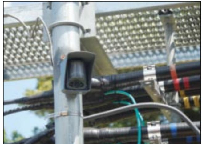
**This camera gives a straight view from the cable tray looking outward, revealing any possible intruders to viewers at the security monitoring center. Metal thieves might be attracted by the copper in the wires shown here covered with green insulation.**
