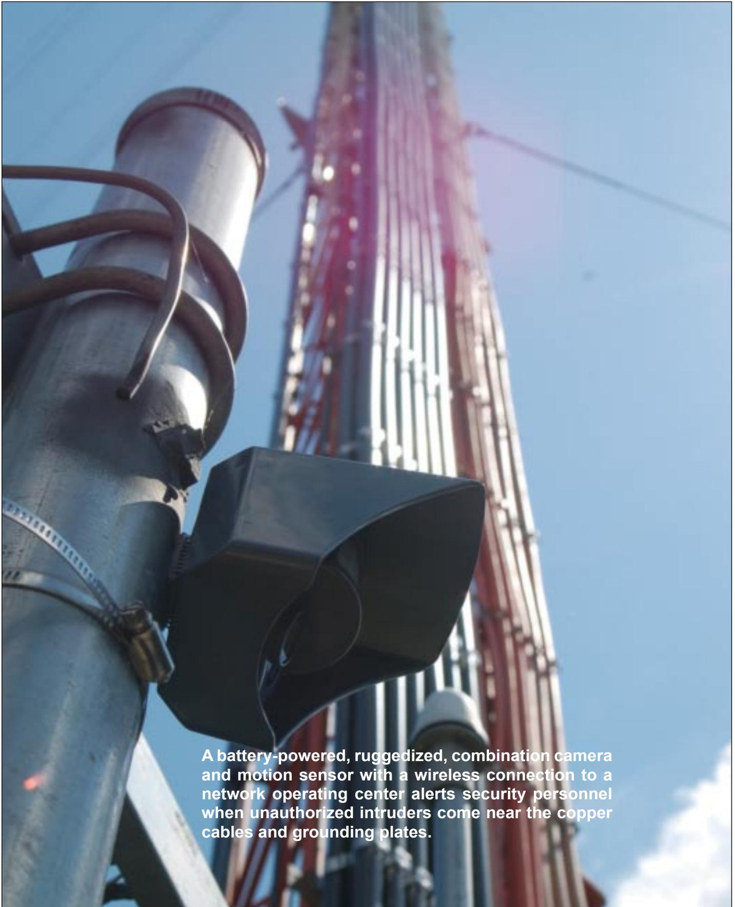
A battery-powered, ruggedized, combination camera and motion sensor with a wireless connection to a network operating center alerts security personnel when unauthorized intruders come near the copper cables and grounding plates.
